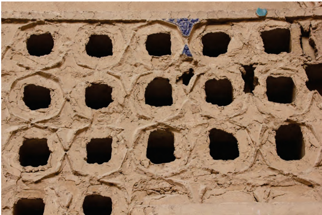
Img. 11: Detail of the grill separating the burial chamber of the Shaykh from the main space of the iwan of the Pir-i Bakran mausoleum: tile shapes and dimensions are visible on the adhesion mortar, which contains some tile fragments.
