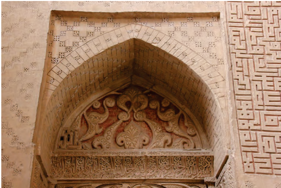
Img. 2: Example of stucco revetments in the Pir-i Bakran mausoleum: south-eastern supporting wall reveals two layers of stuccos from the second and third decorative interventions. (Grbanovic 2018)
