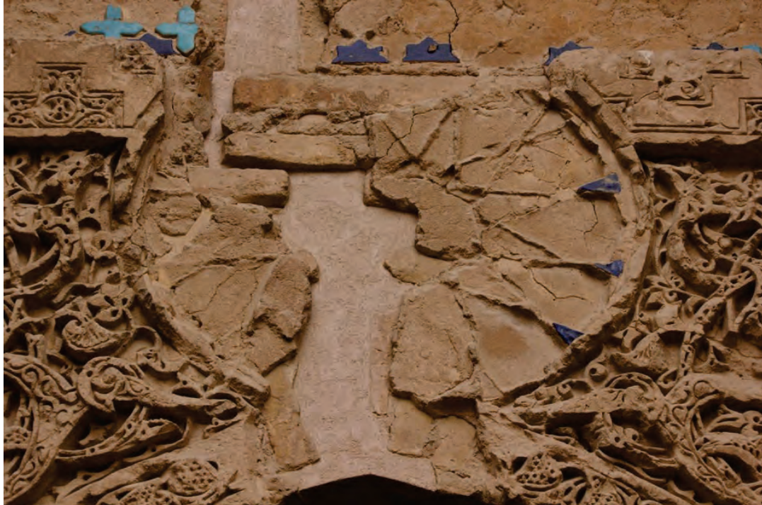
Img. 9: Remains of adhesion mortar for the tile rosettes on the entrance portal of Pir-i Bakran mausoleum's entrance corridor. The mortar retains small triangular glazed and moulded tile inserts. (Grbanovic 2018)
