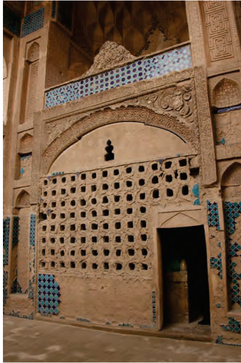
Img. 8: Grill separating the burial chamber of the Shaykh and the interior space of the iwān . The grill retains mortar for the adhesion of tile revetments. (Grbanovic 2018)
